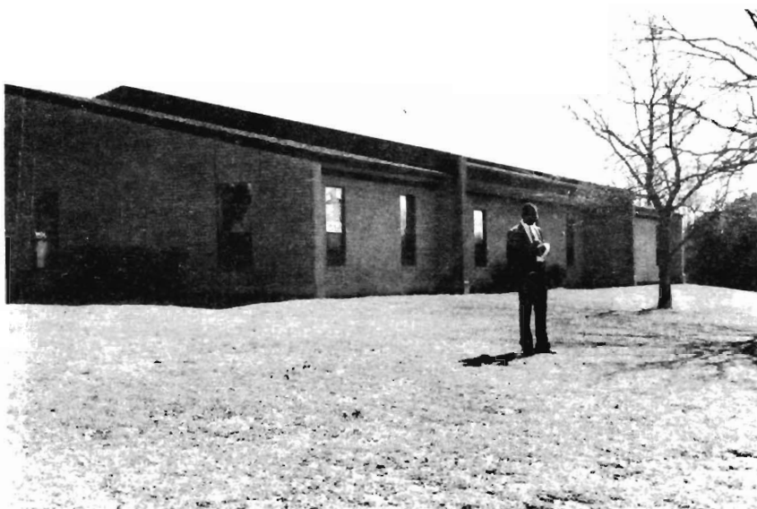
The Mayborn Building of the Vanguard School. It was recently built.
